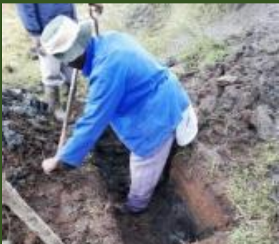
Digging offtake for slotted pipe
